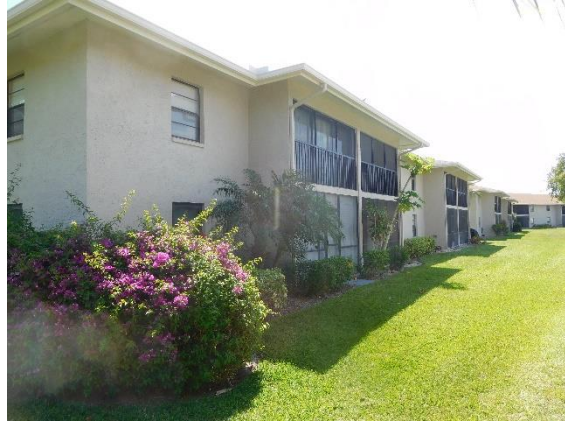
REAR VIEW 8 UNIT BUILDING
