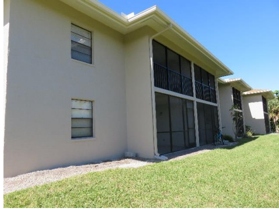
REAR VIEW 7 UNIT BUILDING
